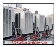
Dirty coils can increase energy use by more than 30%. Additionally, dirty coils can make the compressor work harder and lose up to 30% of cooling capacity. Ideally, air conditioning maintenance should be done twice a year.
